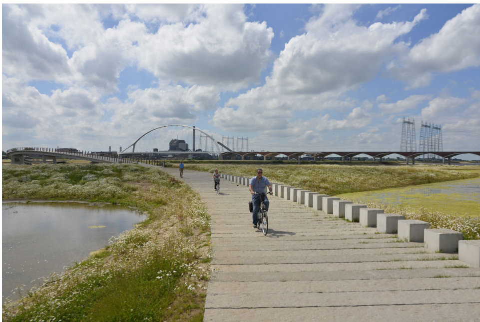
Foto NEXT Architects Zalige Bridge
